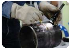
Welding Inspection CSWIP
